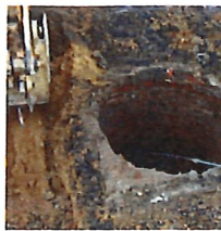
Inlet to Manhole Repair
