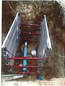
Inlet to Manhole Repair
